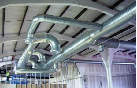
IoT sensors Indoor Air Supply Lines
